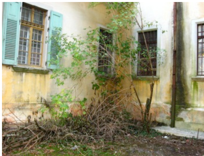
Figure 32: Exterior of the former Kitchen building, September 2011
