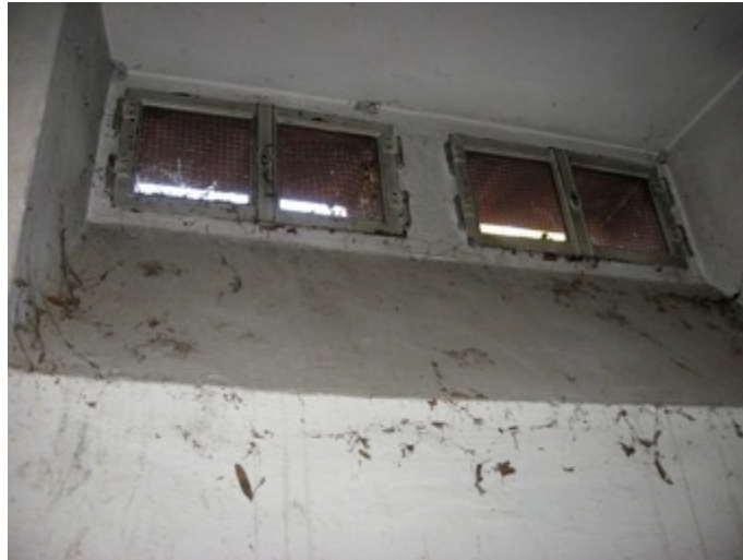
Figure 23: Windows in the basement of Direction building, October 2011
