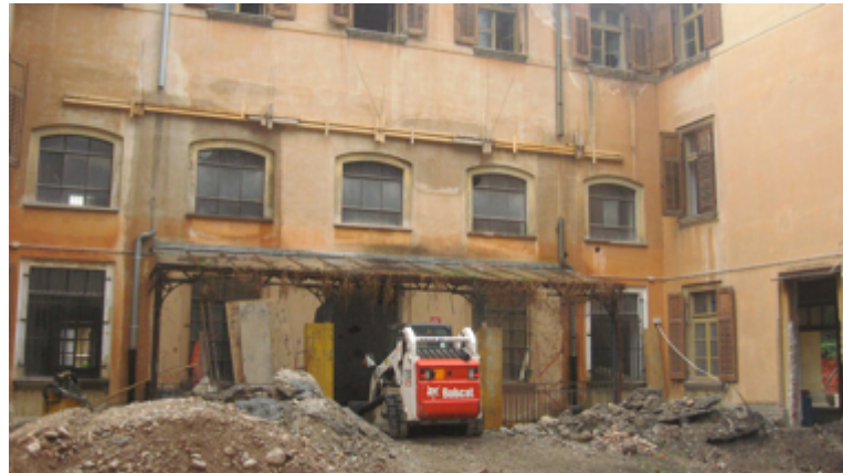
Figure 54: Works on former Kitchen building, July 2013
