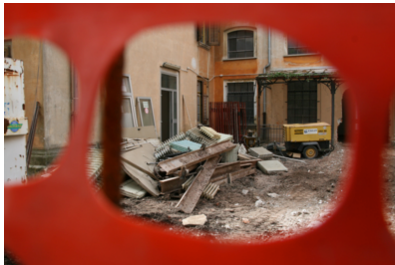
Figure 53: Works on former Kitchen building, April 2013
