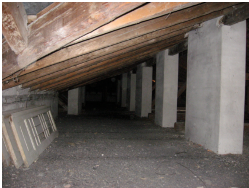
Figure 50: Attic of former Ward B Female, February 2012
