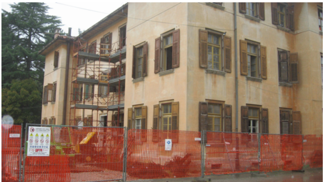
Figure 55: Works on former Kitchen building, July 2013
