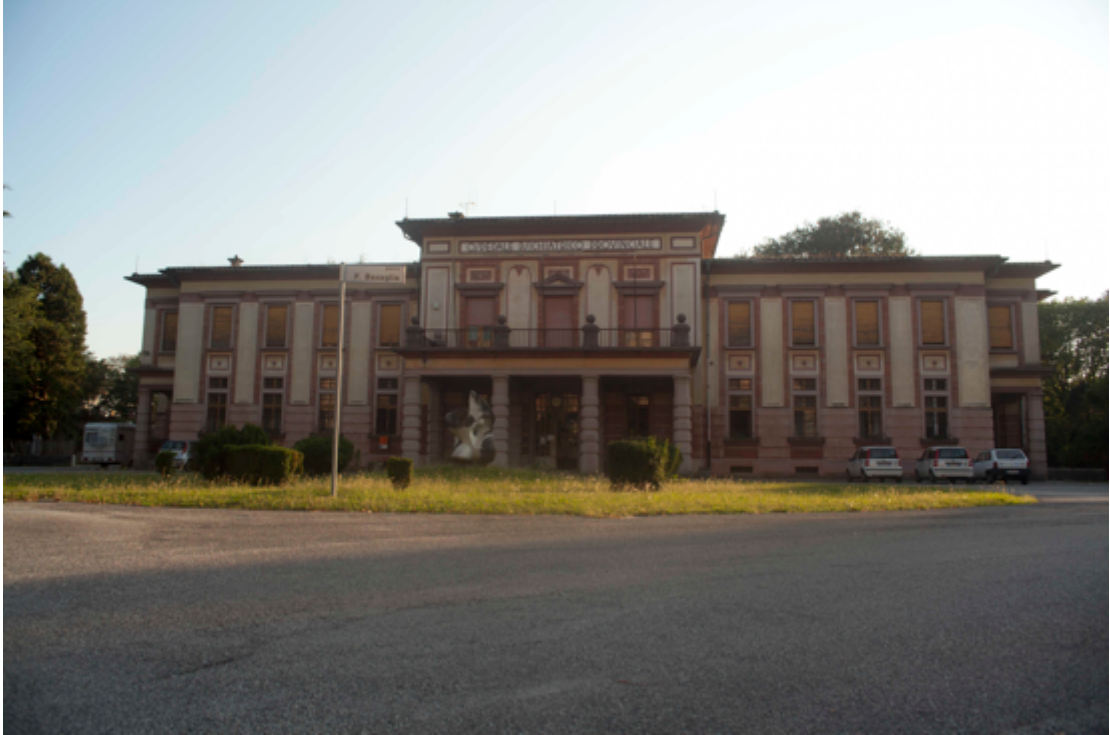
Figure 3: Former Direction Building, October 2011
