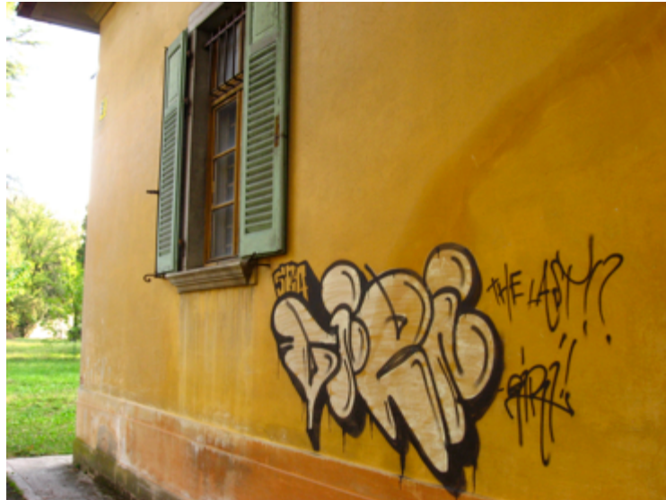
Figure 37: External wall of former Ward B Female, September 2011
