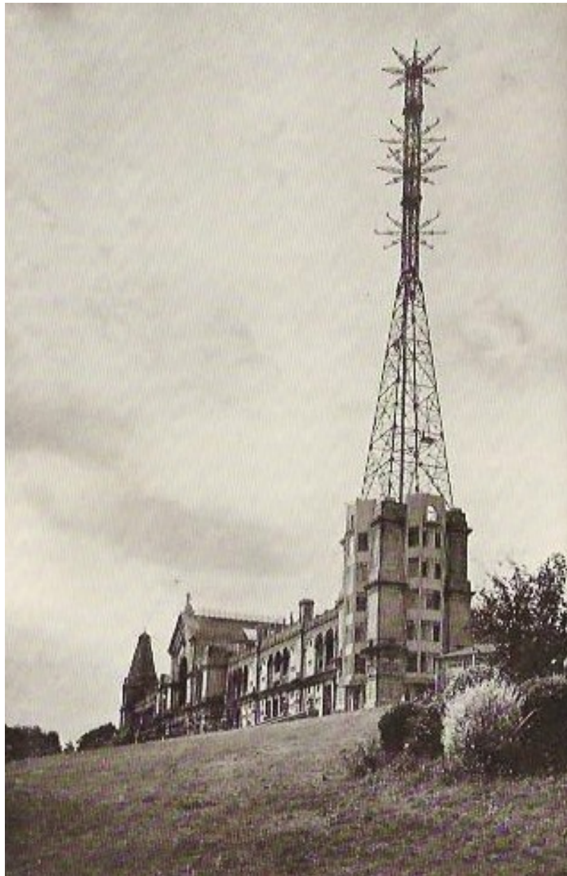
Fig. 2-4. Alexandra Palace Transmitting Aerials, London. Photo by B.B.C. Public Domain.
