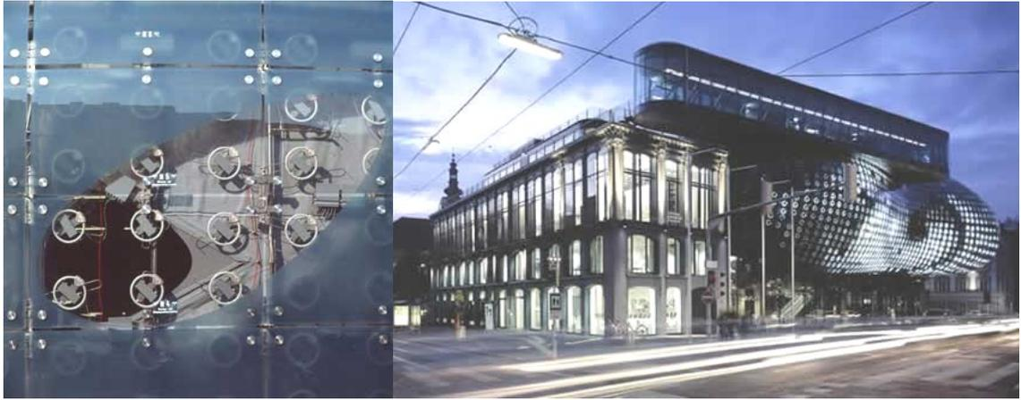
Figure 4.12: *BIX Communicative Display Skin*, Kunsthhaus Graz, façade detail, 2003 and Figure 4.13: The Façade's front view, 2003.
