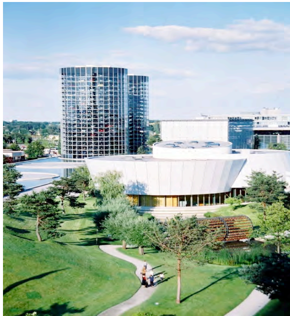
Photograph 6: The Audi pavilion (Autostadt GmbH)
