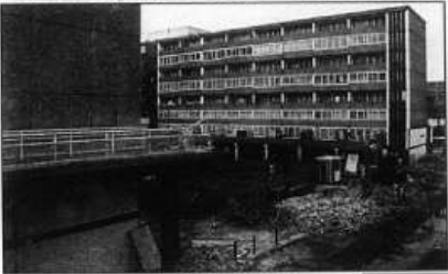
■ Walkways demolition gets underway Photo: TM DICKSON
