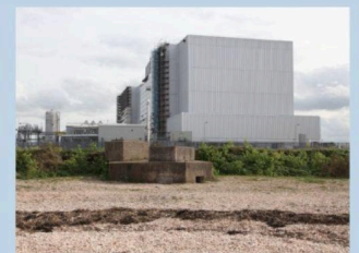
Bradwell A reactor building in the background, partially encased in its weather envelope. A World War II pill box in the foreground.
