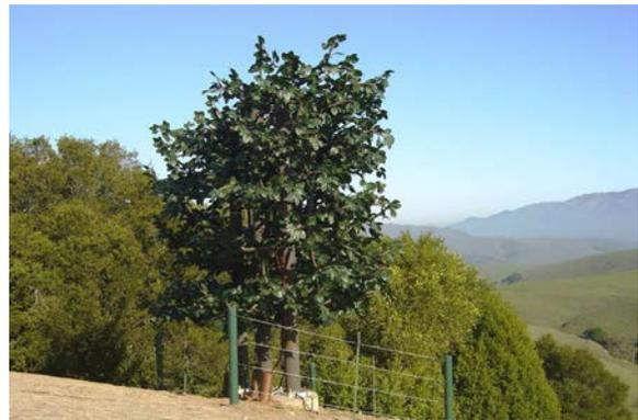
Figure 24 - An 'Elm' concealed cell phone tower manufactured by Valmont Structures
