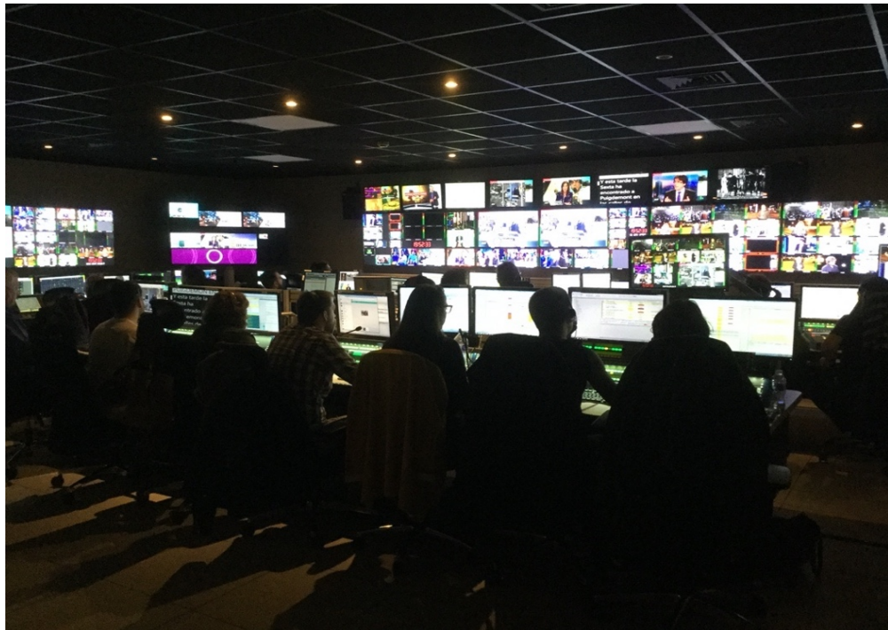
Figure 6-8: One of the broadcast switch rooms at Atresmedia used by La Sexta News programme 58
