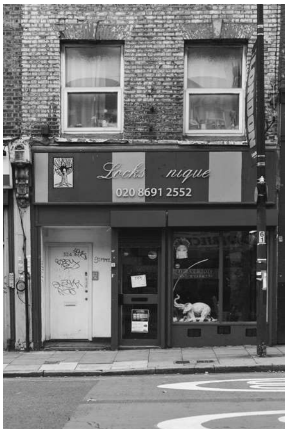
Fig. 3.6 324 New Cross Road
