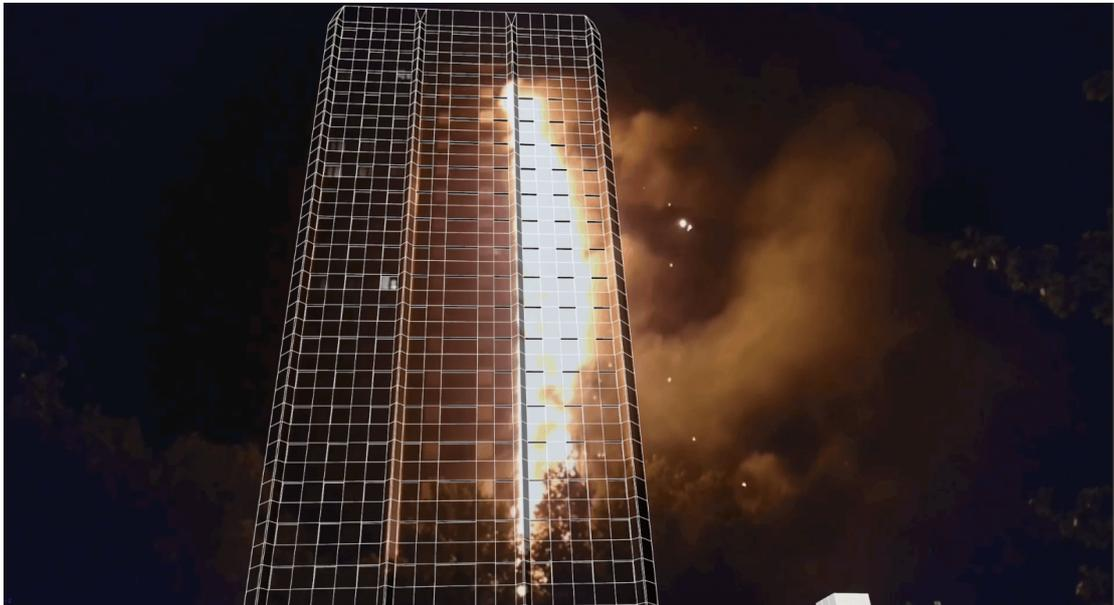
Forensic Architecture, *The Grenfell Tower Fire investigation. Projection Mapping – 1*. Video footage of the fire is ‘motion tracked’, and mapped onto a wire-frame model of Grenfell Tower. © Forensic Architecture, 2019.
