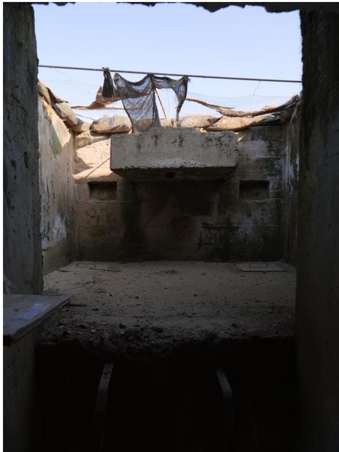
Inside the berm / tank trap.
