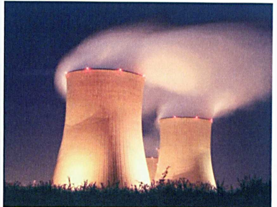
S402 Cattenom Nuclear Power Station, France.
