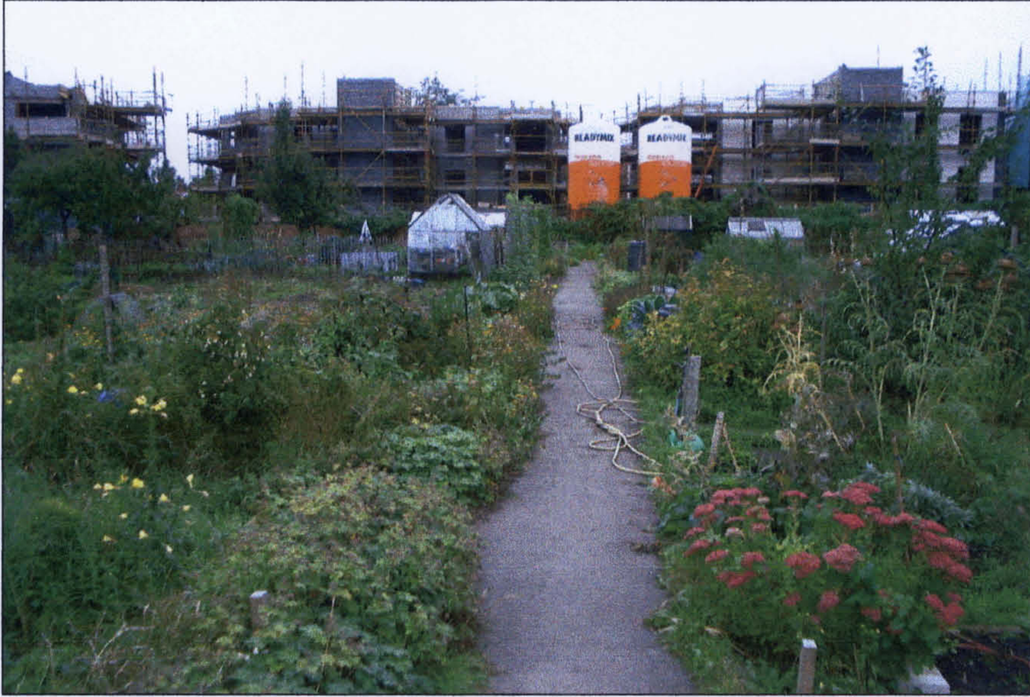
Figure 6.3 Apartment Development Adjacent to Allotments
