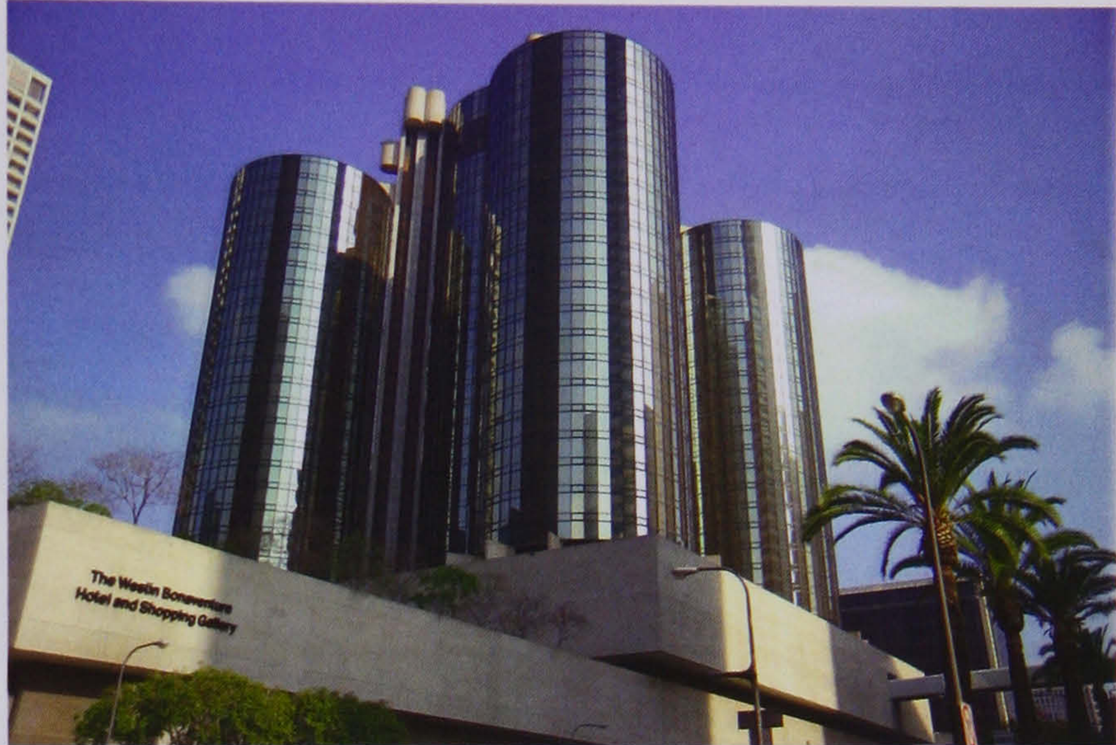
3.2 - The Westin Bonaventure Hotel (exterior view).
