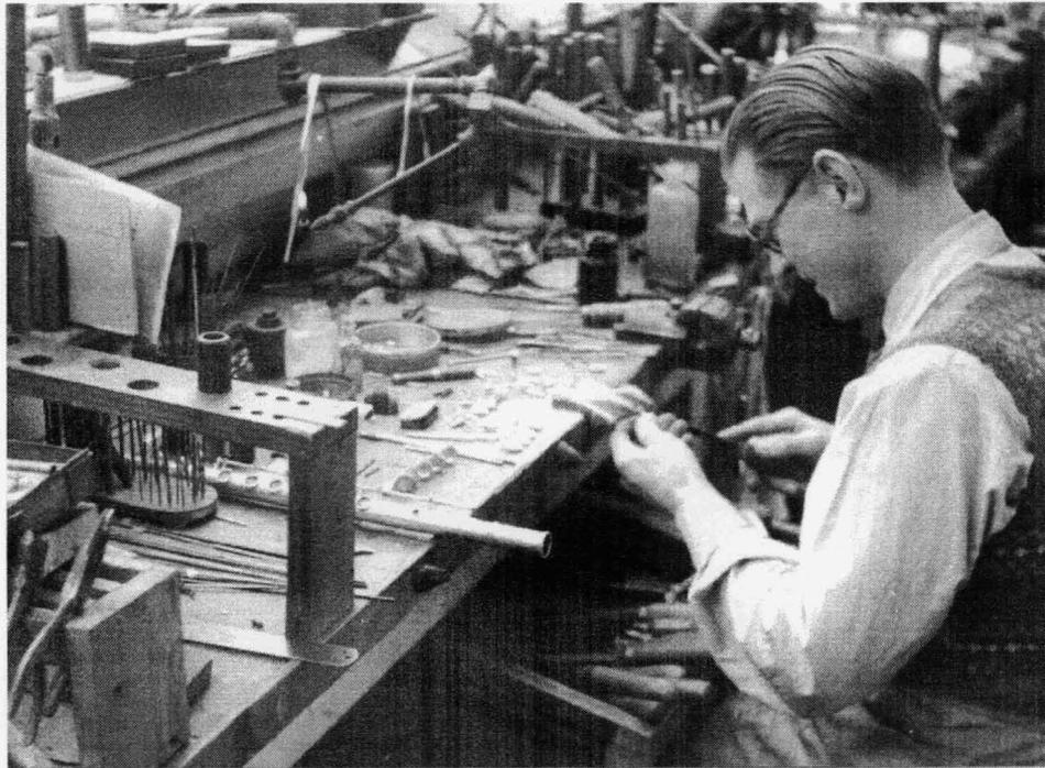
Albert Cooper at his workbench. Note the gas burner, which appears to be one of the same burners shown in the 1913 photographs. The workers were expected to solder the keywork on their flutes using the gas burner, enhancing the flame with a blowpipe held in the mouth. Photograph by Roger Charters.
