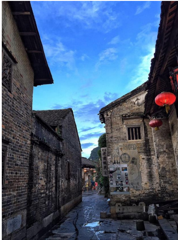
Figure 18. A photo from Tianran Street where the Relevant Hotel stands. No electricity wiring like this should appear on a main street. Source: photo credit by the owner of the Relevant, July, 2015.
