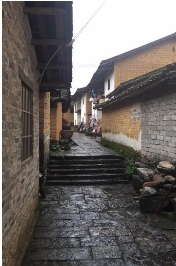
Figure 19. A photo from the back of Tianran Street. Electricity wires can be seen under the eaves and across the street. Source: photo credit by the author, July, 2017.
