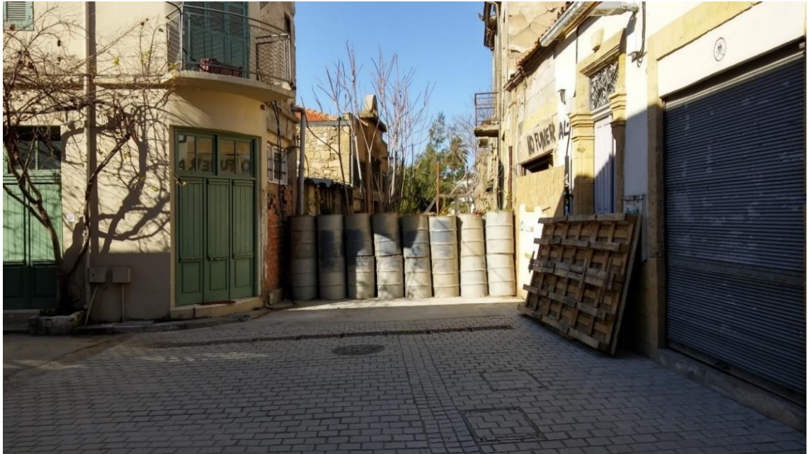
Figure 5: As the line cuts through the old town, behind the oil-drums the abandonment is evident. In the front, restored building facades and streets. Photo by author, 2016.
