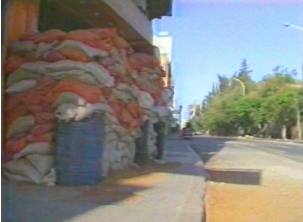
Figure 3: Sand bags used on the ground floor of a domestic building in Beirut to protect the civilians living there from the Lebanese Civil War, 1989. Courtesy and copyright of BBC News.
