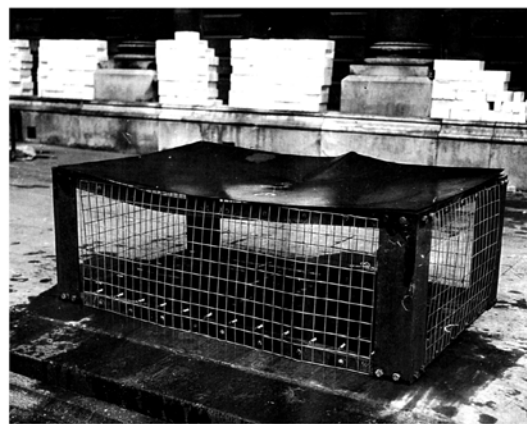
Indoor Air Raid Shelter. Tests carried out by the Research and Experimental Department. Flat-topped shelter Type T. This shelter was first tested by dropping a heavy block of concrete weighing 350 lbs from a height of 6 ft above the top. The flat top was only dented. The shelter was then subjected to a second test in which a floor weighing 1,800 lbs and pivoted at one side was dropped 6 ft 6 inches and with a swinging action so that it struck one top edge of the shelter as it fell, simulating the manner in which the floor of house usually collapses. The steel angle at the top edge was bent.
