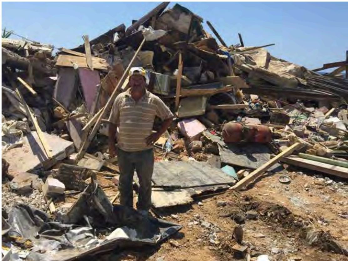
Figure 39: Fishermen standing in front of their homes on the Beirut coast, destroyed by the Lebanese government to allow for a new luxury development. Photographs by Habib Battah, 2016.
