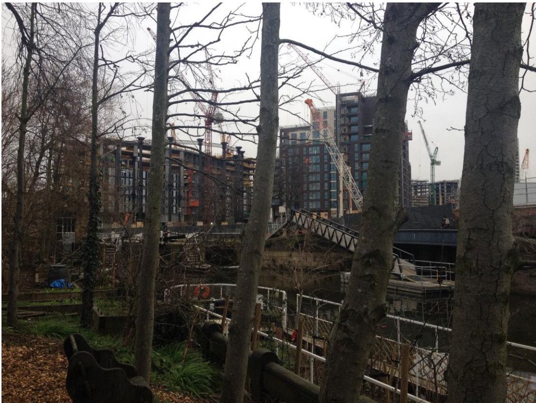
Figure 14: Camley St. canal side, with the surrounding building works in progress.
