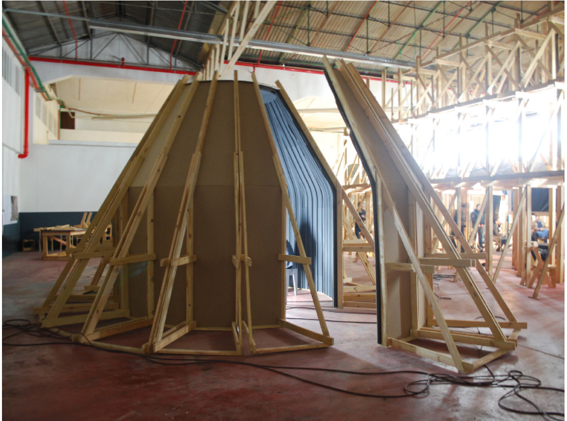
Fig. 4.1. Radio Sonores installation at ASA factory
