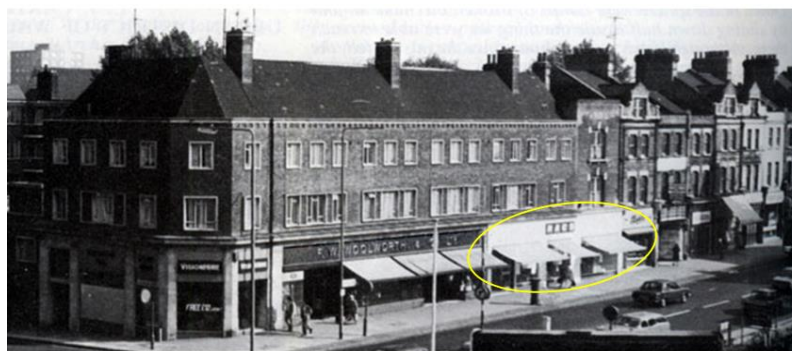
Figure 7.3: The New Cross Library building when it was a grocery store, highlighted to the right of Woolworths, early 1960s following post-war reconstruction. (Image: The Woolworths Museum, 1960)
