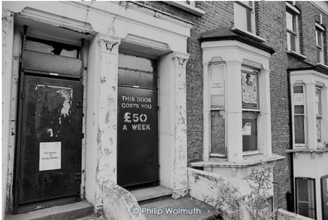
Image 4 Boarded up houses on Walthamstow Avenue, W9.
