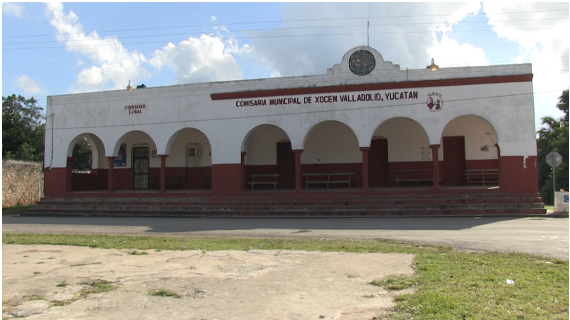
Figure 3: Municipal administration building, Xocén
