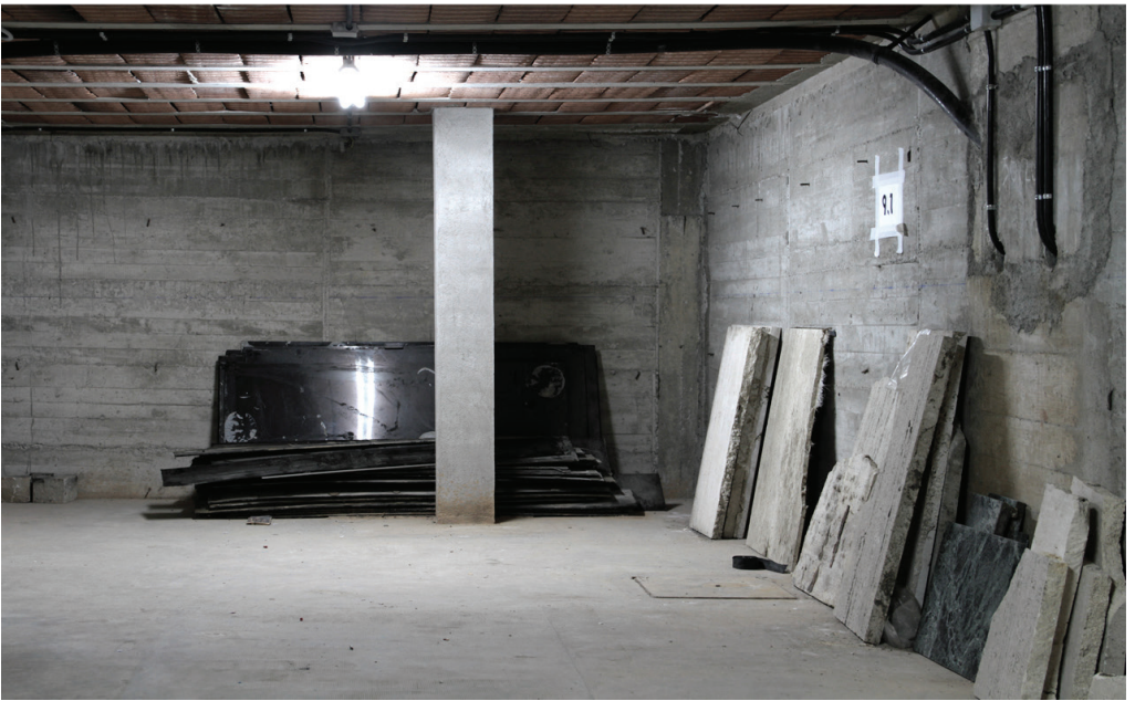
FIG. 6.1 Barcelona Pavilion, above and below ground (photos and composition: Andrés Jaque, 2012)
