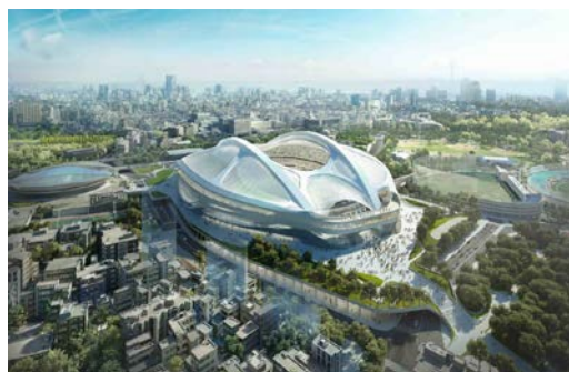
Figure 1 Zaha Hadid’s revised design of the Tokyo Olympic Stadium
