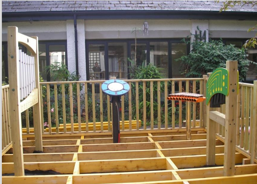
Photograph 16: The care home's musical garden (under construction)
