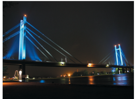
New Railroad Bridge, Belgrade
