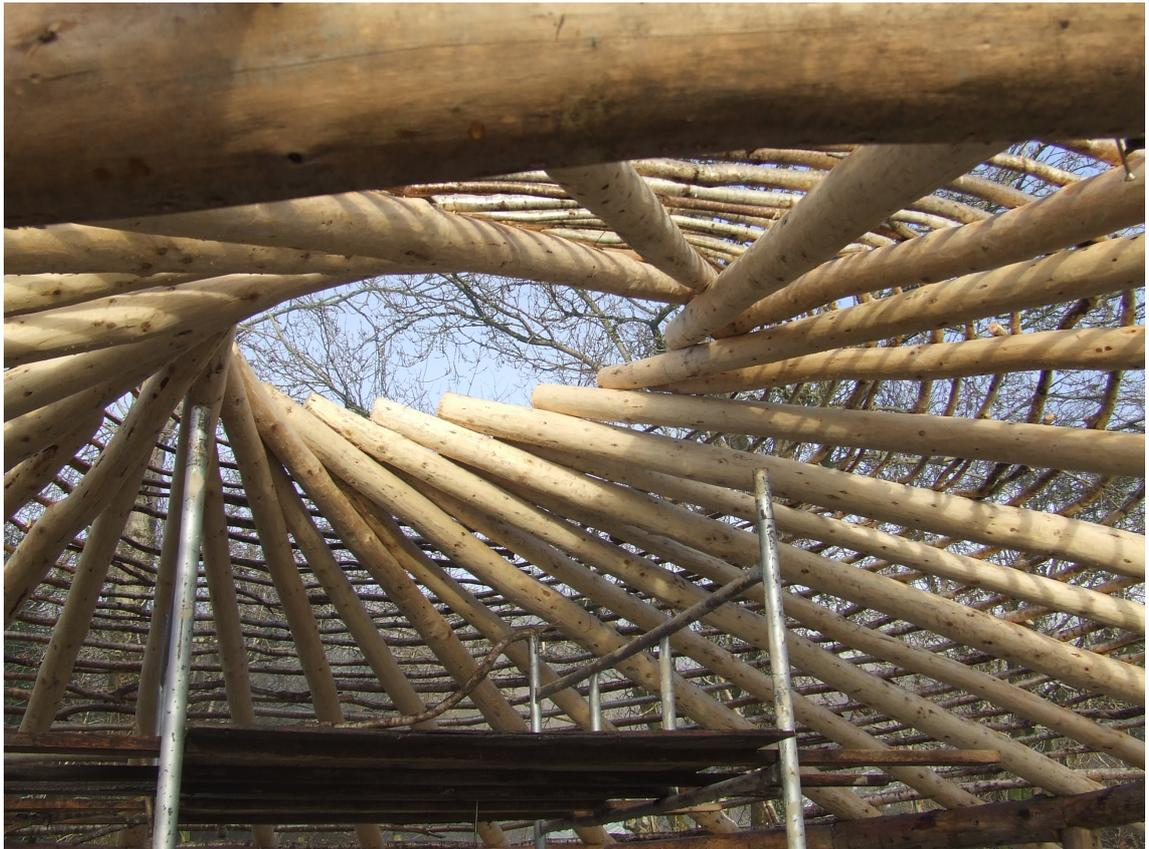
Figure 5 Photograph showing a reciprocal roof frame (c) Forde
