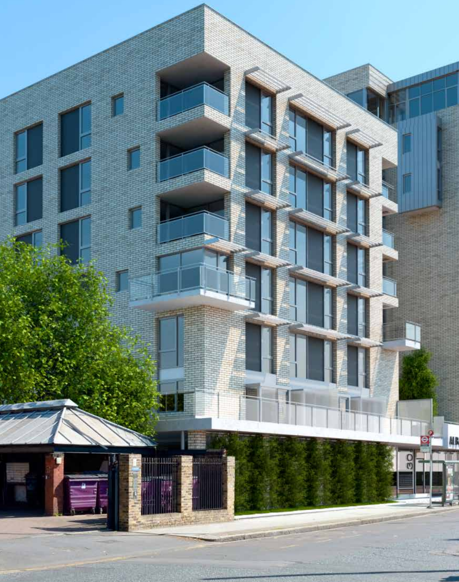
Burgess Terrace, Aylesbury Estate, Southwark
