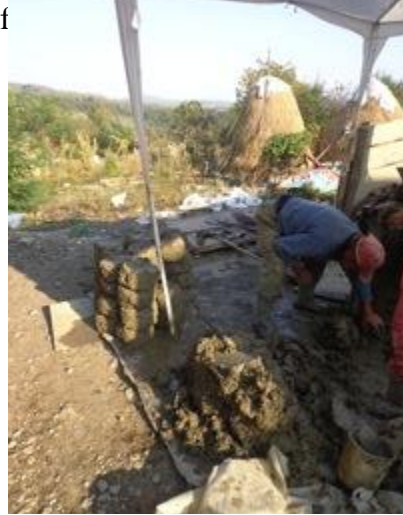
Fig.7.11 Preparation of clay for mixing and moulding (right)
